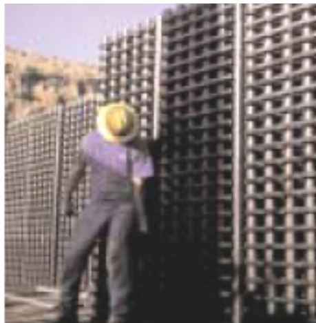
Left top: Product and installation of watershed storage units from Invisible Structures Inc.
